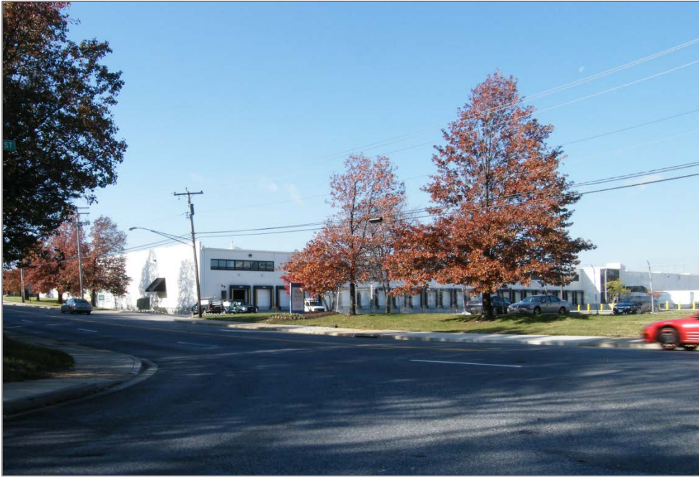
Figure 4. 3636 Pennsy Drive, south and east facades.
