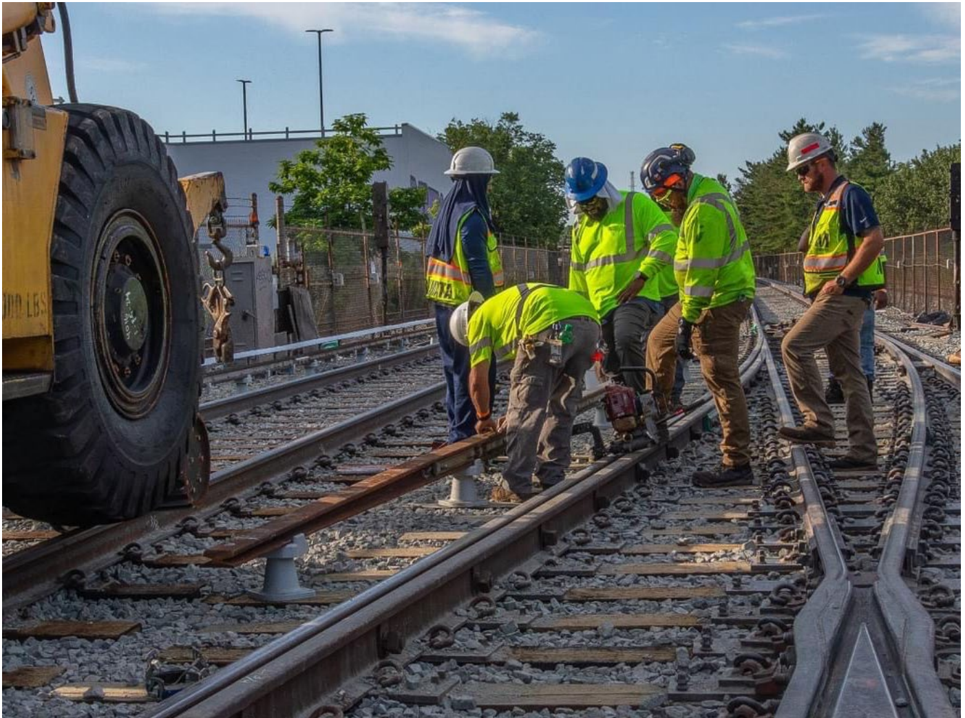
Pictured: Metrorail workers performing necessary track rehabilitation
