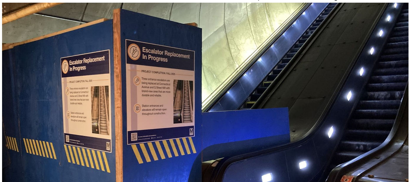
Pictured: Escalator replacement in progress
