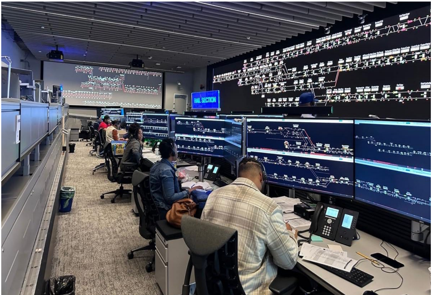
Pictured: Metro Integrated Command and Communications Center (MICC)
