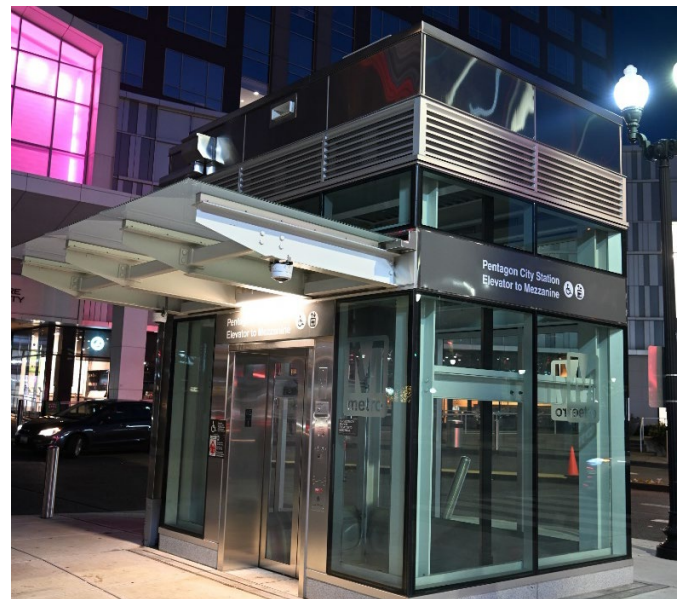
Pictured: Pentagon City Metro Station elevator installed in 2025
