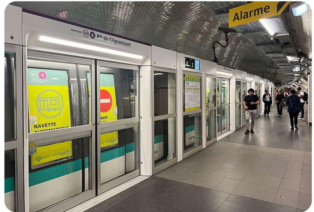
Paris Metro: Line 4 Platform Screen Door Testing
