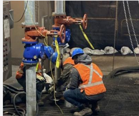
Drainage Pumping Station Work
